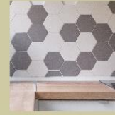
DADO CERAMIC TILES 600 MM ABOVE THE COUNTER
